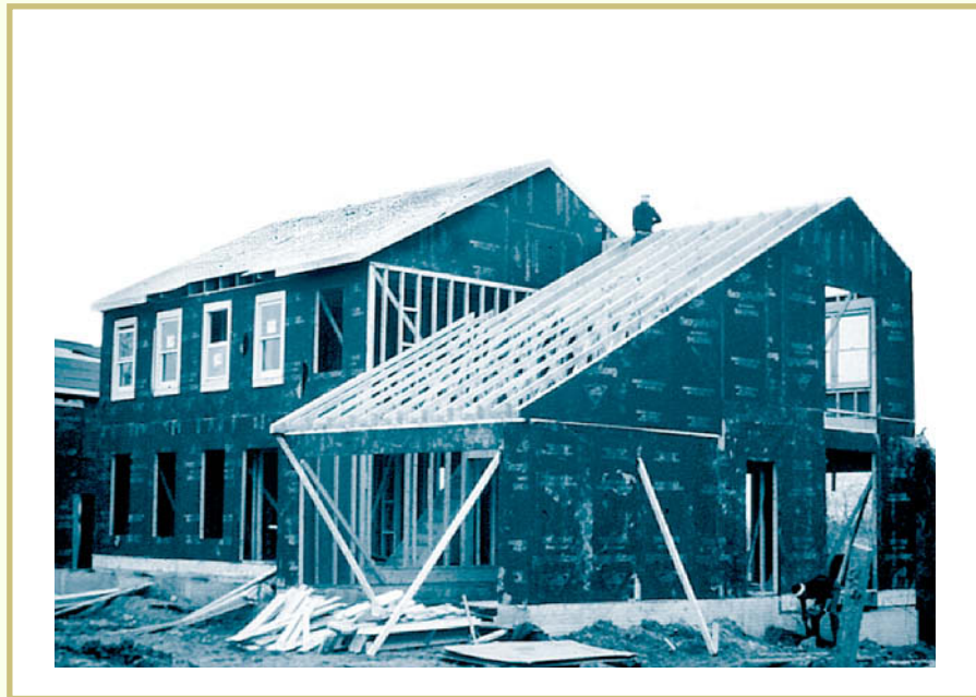
FIGURE 2 —This figure illustrates the process of rough carpentry.
